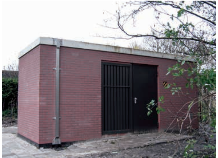
Image of an area point of presence, used for aggregating thousands of Internet connections whilst being protected with a simple lock
